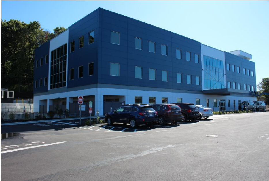
Fallon Health's newest PACE site located in Worcester, Mass.
